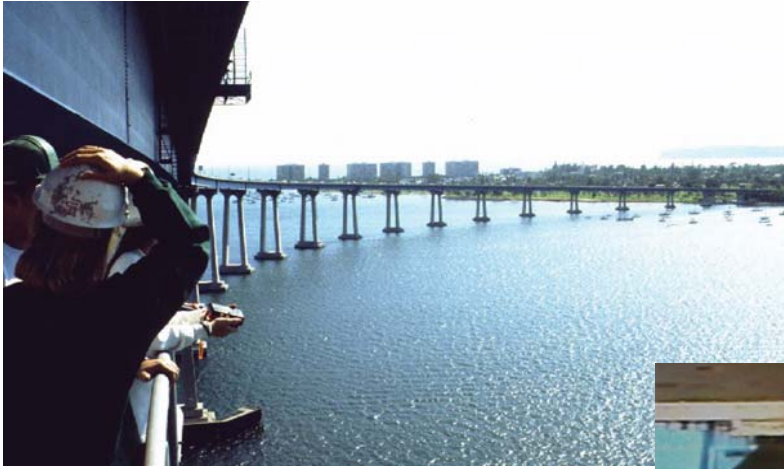
Coronado Bridge, one of three major toll bridges in California that may be seismically retrofitted with huge bearings and dampers.
